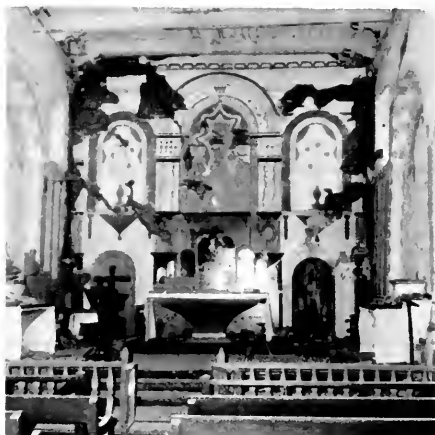
Photo 1. Photo showing damage to non-reinforced adobe walls in the interior of the chapel of San Fernanda Mission, originally built in about 1806.
